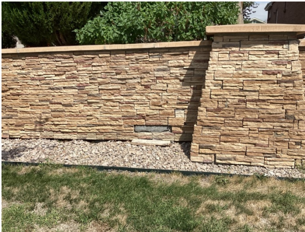
Missing masonry stone at the masonry perimeter wall
