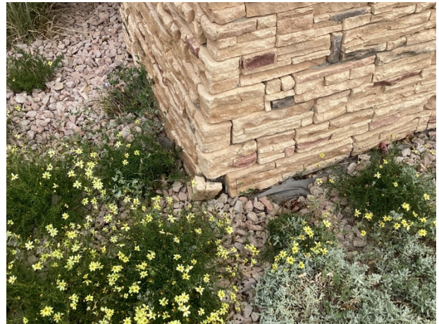
Masonry stone damage
