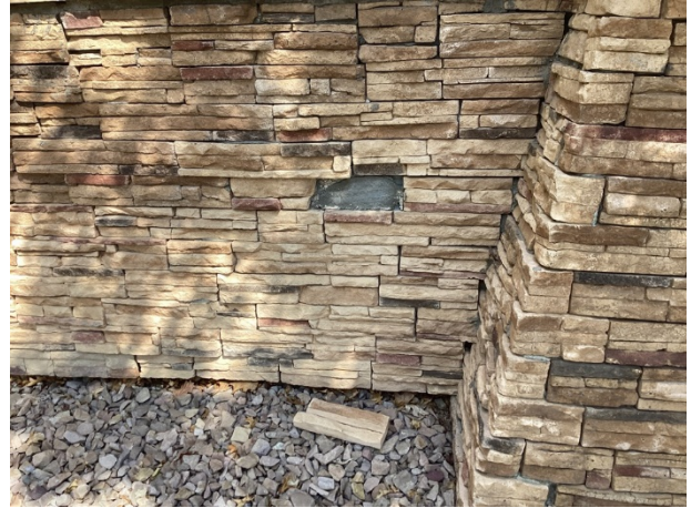
Missing masonry stone at the masonry perimeter wall
