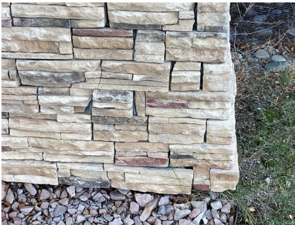
Masonry stone cracks and loose stones
