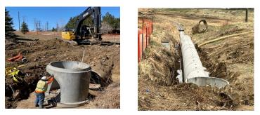
detention ponds located in the Xcel easement area. The project includes extending the concrete storm drainpipe at the pond inlet by approximately 80 feet. Once in place, the drainpipe will be buried to fill-in the trench running alongside the City's pedestrian and bicycle path. This will eliminate a steep dropoff along the path and return the surrounding area to a consistent and much safer grade. Pond
